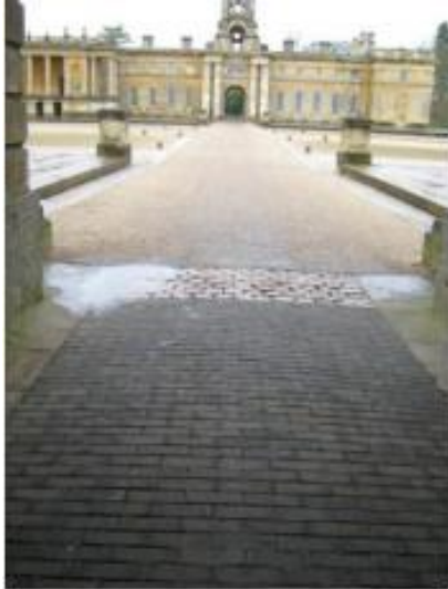
Example of uneven surface
